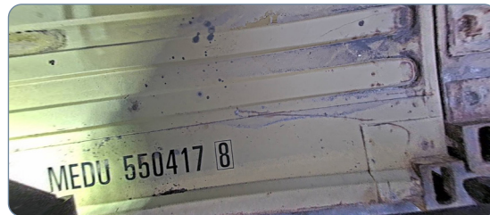
4 Container ID from the roof
